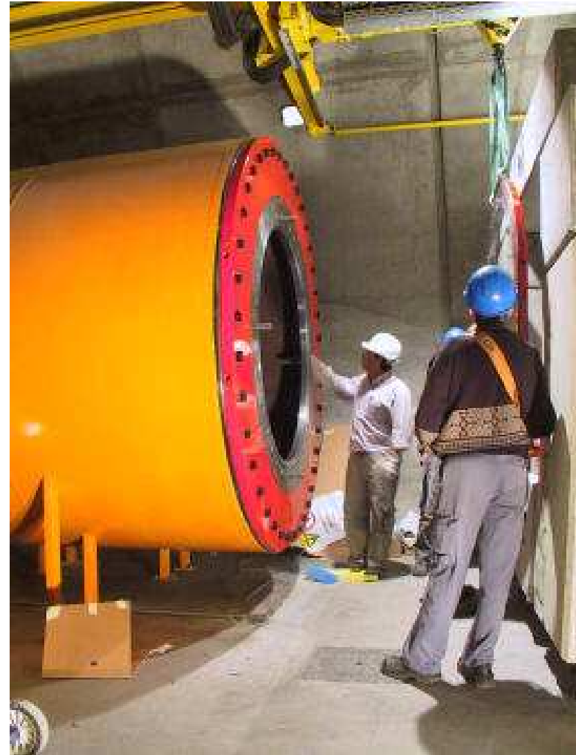
Reflector and decay-tube installation
