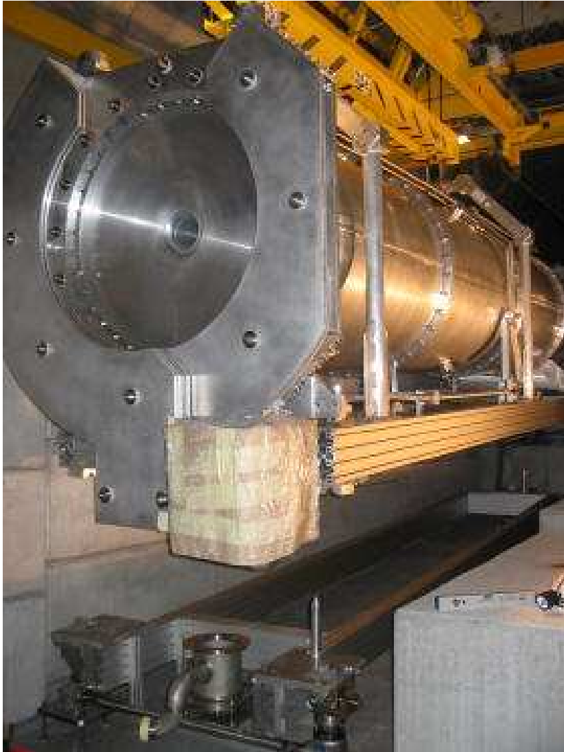
Reflector and decay-tube installation
